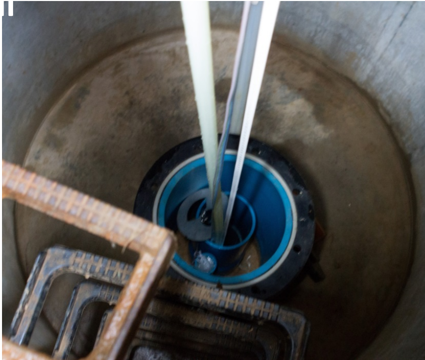
View borehole (ca. 10'000L)
